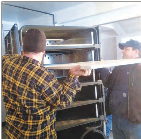
Boulangerie co-owner Zachary Tyson, left, gets help placing deck stones into the bakery’s oven from Bill Lawson of Empire Baking Equipment. Before the stones went all the way in, Lawson and Tyson gave each one a little leveraged jolt to crack them.
